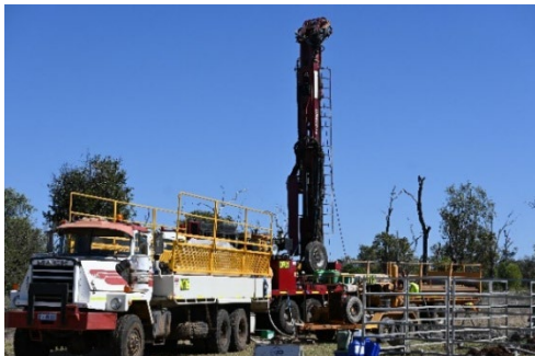
Plate 1 Exploration Drill Rig On-site
