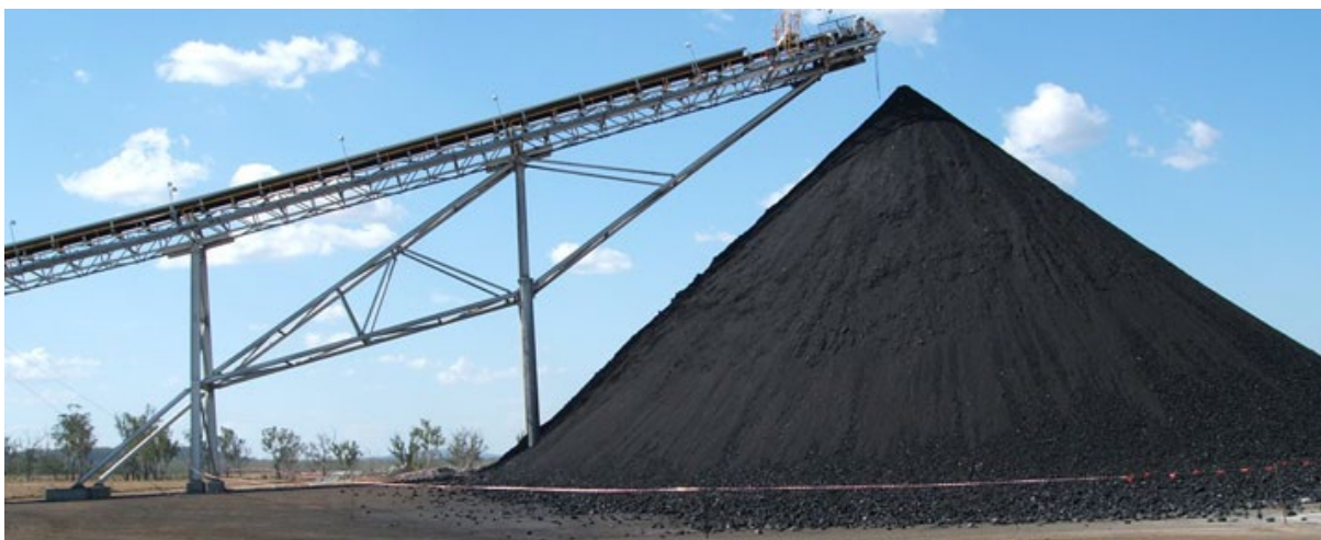
Plate 5 Example of a Drift Conveyor and ROM Stockpile (Source: Nepean, 2006)
