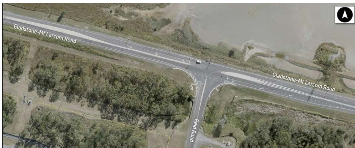
Figure 7 Existing Gladstone-Mount Larcom Road / Reid Road Intersection, Yarwun
