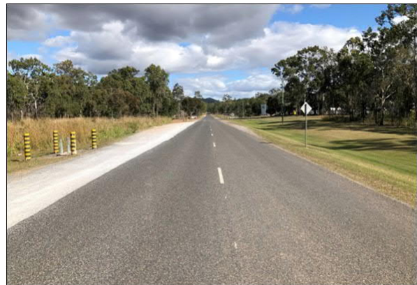
Figure 6 Reid Road Configuration (Looking South)
