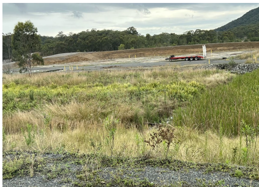
Photo 7: View across the Project site – road upgrades along Euroa Circuit are currently being undertaken.
