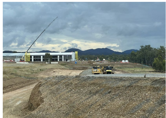
Photo 6: View from the corner of the Project site towards FFI's Electrolyser Manufacturing Plant. Euroa Circuit currently subject to upgrades.
