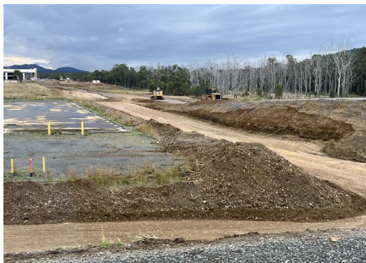
Photo 5: View from a stormwater detention area over the Project site, towards FFI's Electrolyser Manufacturing Plant.
