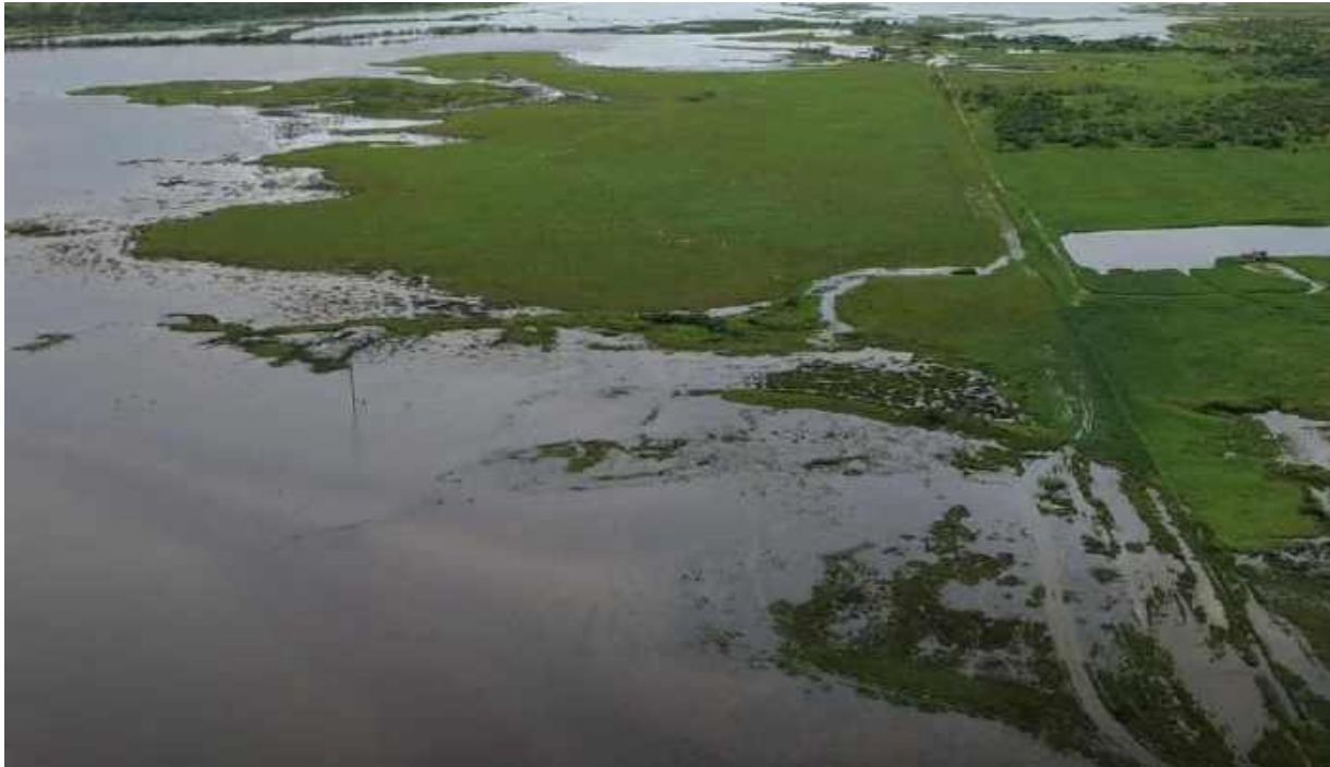
Figure 4-1 TCC Drone image of the site during the February 2025 flood event.
