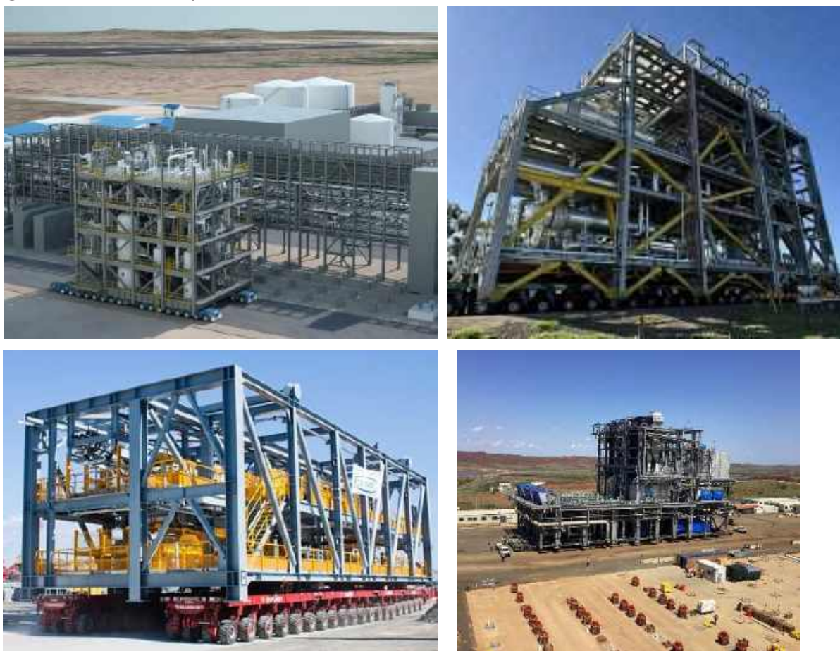
Figure 2: Module Transport to Site
