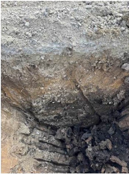
Plate 2: Typical soil profile to 1.2 m BGL, Gravel fill, with brown clay fill and underlying black Clays.
