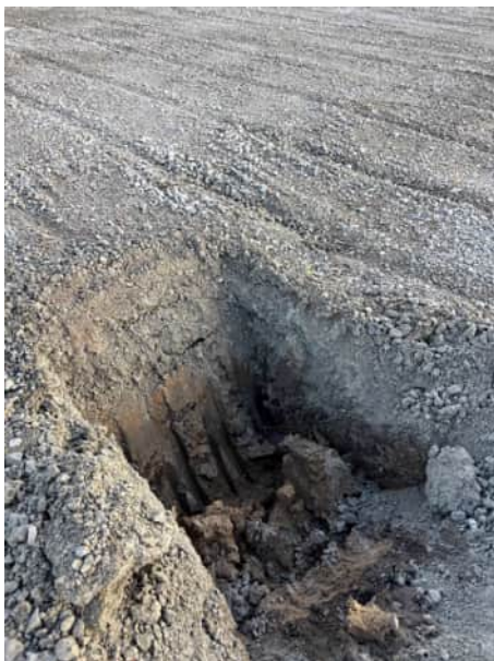
Plate 1 Bore hole highlighting the extent of the gravel fill
