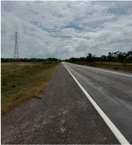
Figure 8 Townsville Port Access Road / Access 2 intersection – looking north
