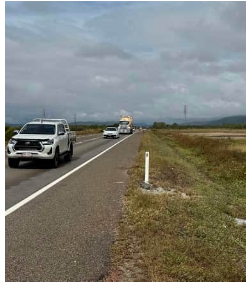
Figure 9 Townsville Port Access Road / Access 2 intersection – looking south
