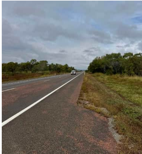
Figure 12 Townsville Port Access Road / Access 3 intersection – looking south
