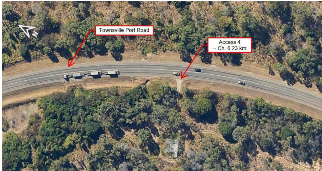
Figure 13 Townsville Port Access Road / Access 4 intersection – aerial view
