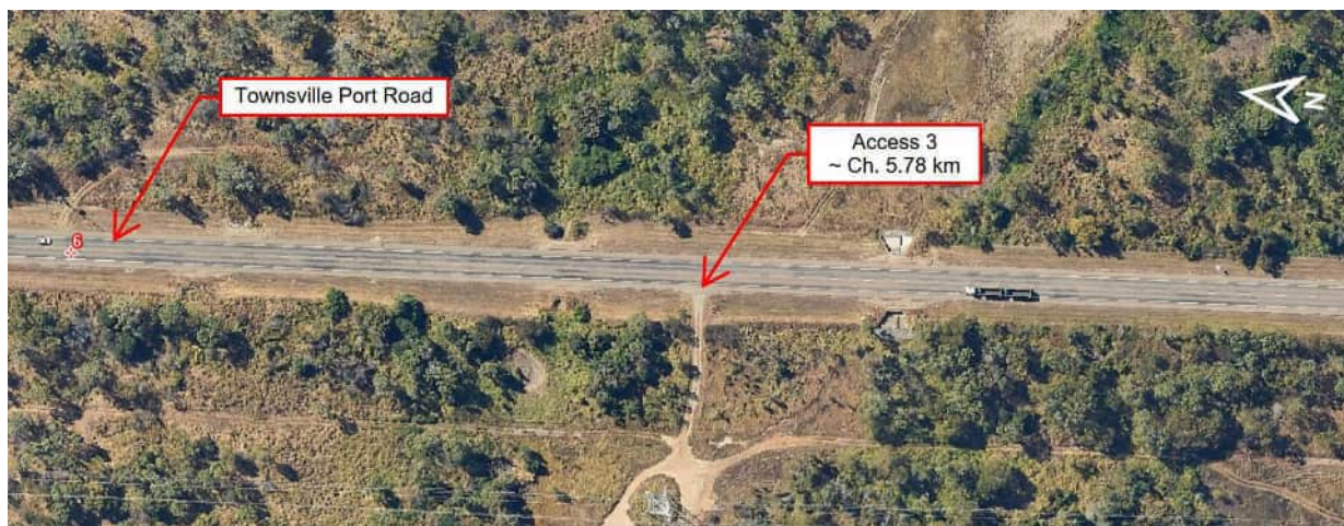
Figure 10 Townsville Port Access Road / Access 3 intersection – aerial view
