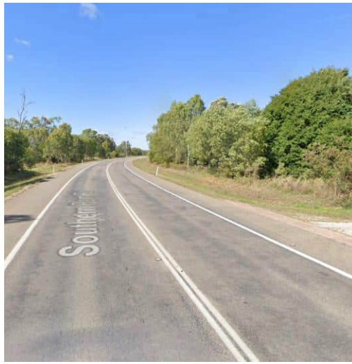
Figure 15 Townsville Port Access Road / Access 4 intersection – looking south [Source: Google Street View]
