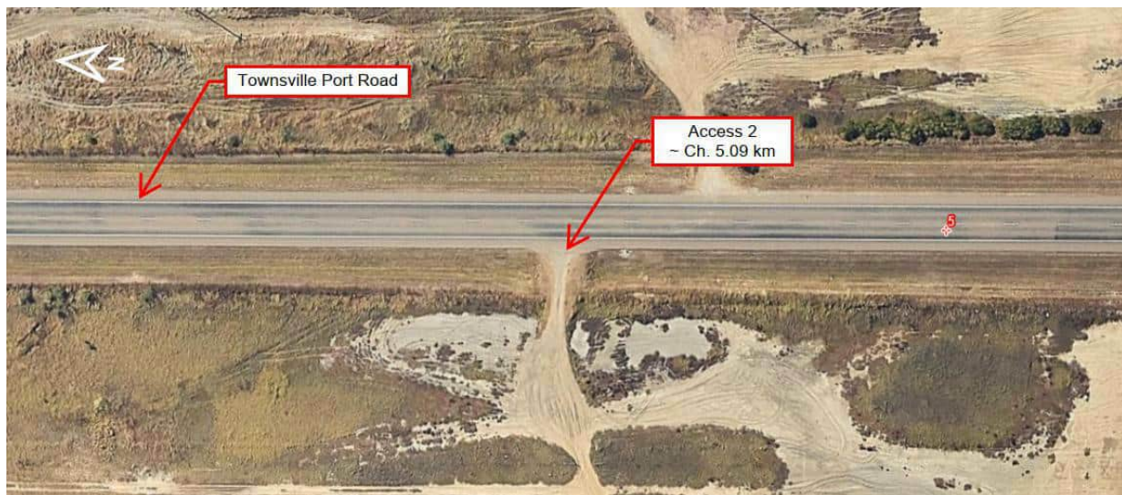
Figure 7 Townsville Port Access Road / Access 2 intersection – aerial view
