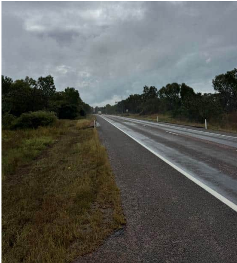
Figure 11 Townsville Port Access Road / Access 3 intersection – looking north
