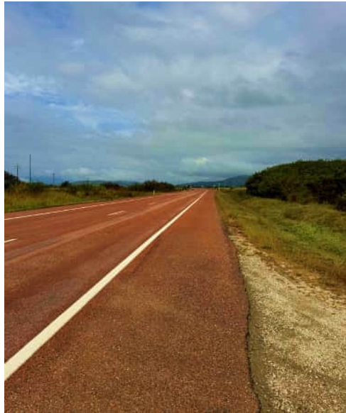
Figure 6 Townsville Port Access Road / Access 1 intersection – looking south
